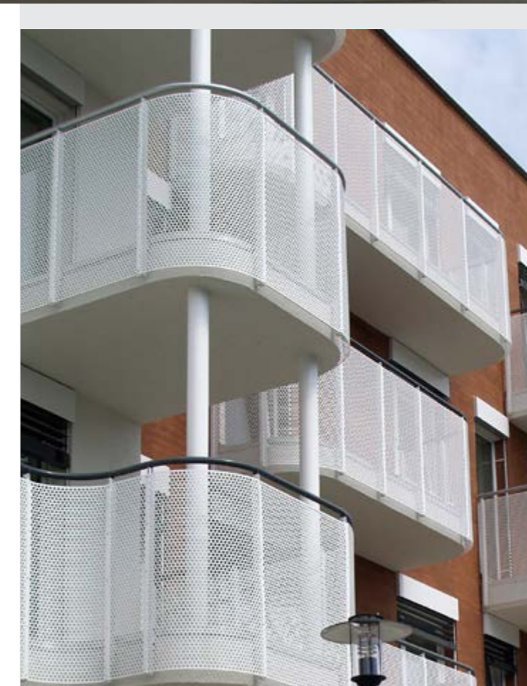
Material used: Railing filling Type: perforated sheet / round holes Rv 20 - 28 Material: pregalvanized steel painted
