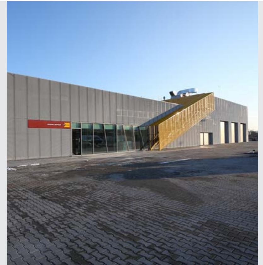
Material used: Facade Type: expanded metal / diamond mesh MR 165 x 55 x 20 x 2 mm Material: aluminium painted
